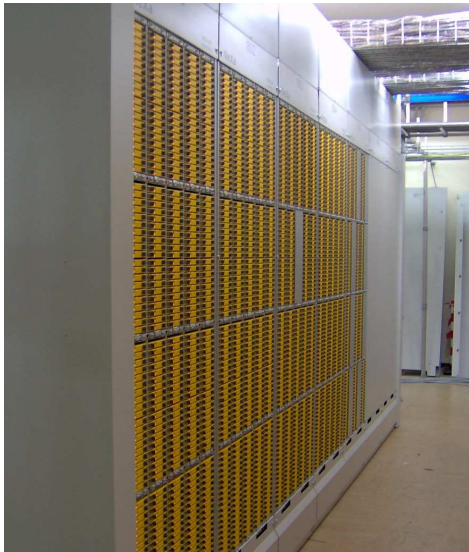
NeXa in a Central Office (CO) solution
